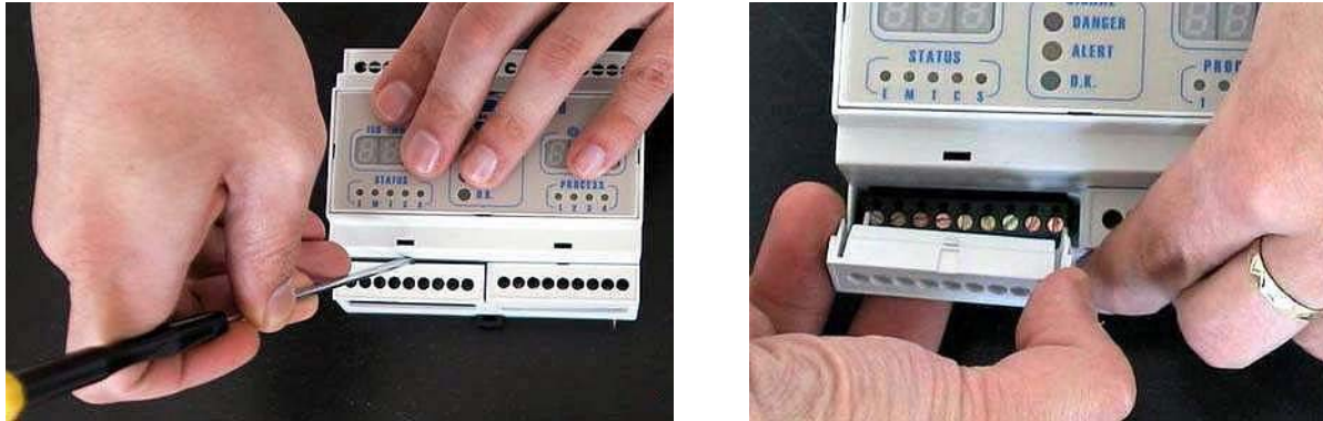
Fig. Removal of the terminal connector covers
